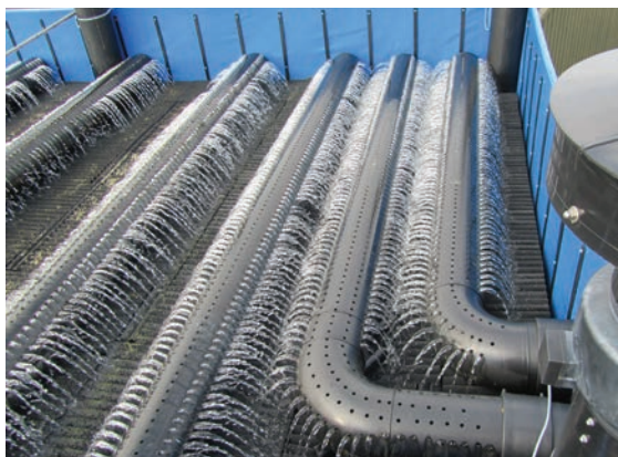
Figure 17. Removal of carbon dioxide for pH regulation. Two different filter types for deaeration of carbon dioxide at an RAS facility. The systems increase the surface between water and air so that carbon dioxide can evaporate to air from the water in a gaseous form, thereby increasing the pH of the water.
