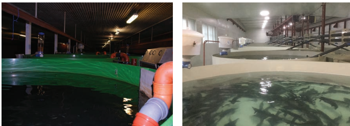
Figure 15. Land-based production systems with recirculating water, RAS. (A) Swedish farming of perch (B) and sturgeon.
