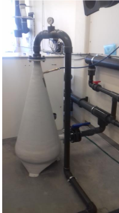
Figure 8. Oxygen cone in Klaipeda shrimps InnoAquaTech pilot farm. Photo: T.Kulikowski/NMFRI
